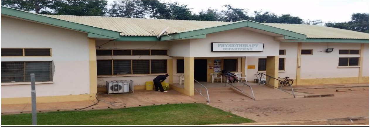
Rehab Dept of KATH Hospital, Kumasi, Ghana
